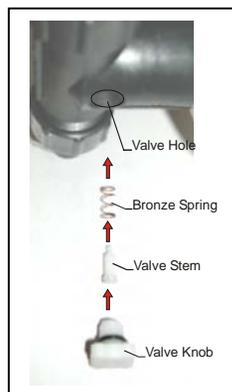
Photo above shows detail of vacuum relief valve for foam bottle. The vacuum relief valve knob does not change the concentration of foam, it only keeps the foam bottle from collapsing as the foam is drawn from it.
